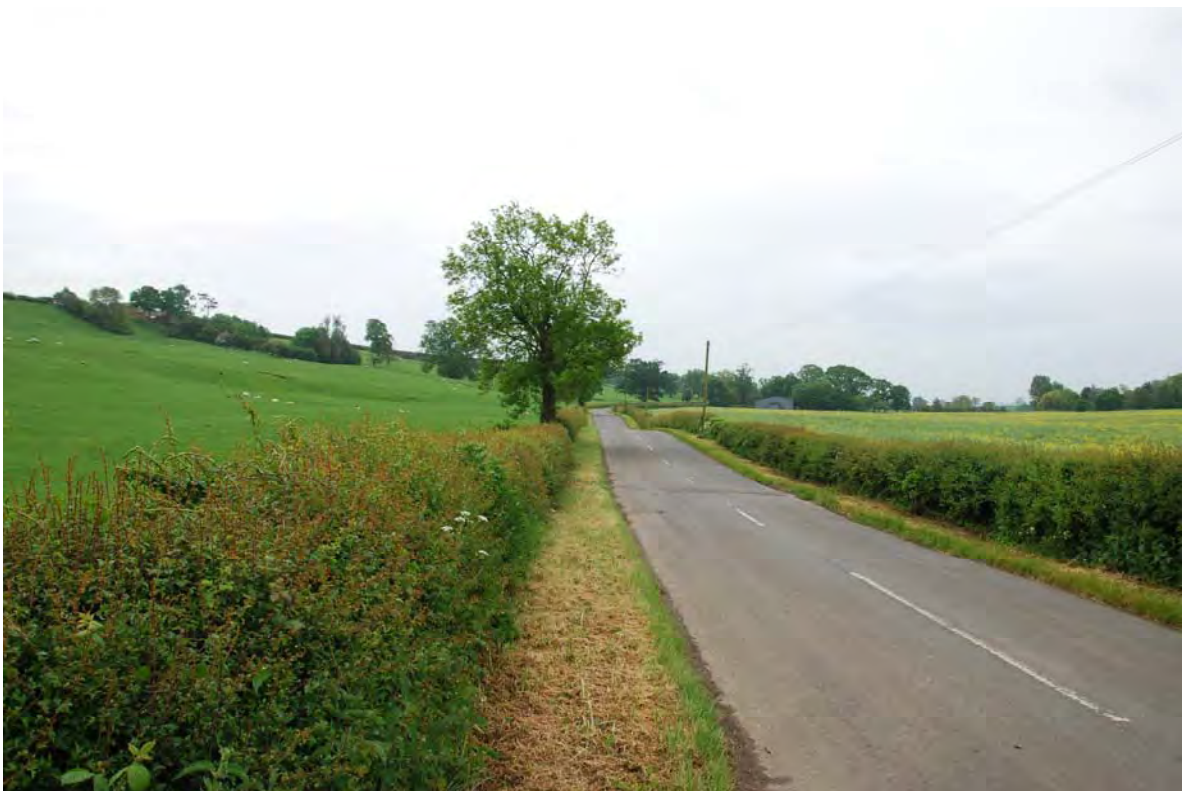
Road with trimmed thorn hedges running along foot of steep slope near the edge of the SLA
